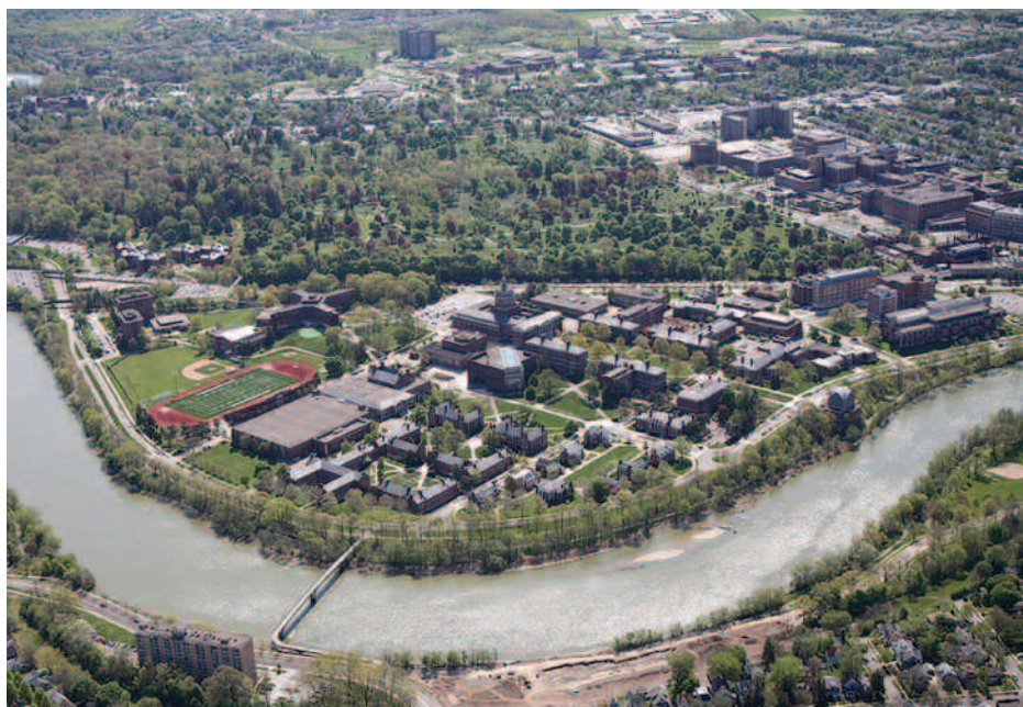
The Genesee River winds along the University of Rochester's main campus, which, together with the adjacent Medical Center Campus (at right), is served by the new low-temperature hot water district heating system.
